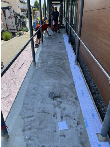
Triflex_Treppe Raika Schwand_05.jpg
