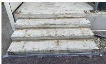
Triflex_Treppe Raika Schwand_02.jpg
