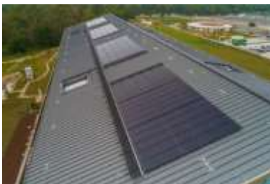
Zambelli RIB-ROOF_PV- Anlagen_06
