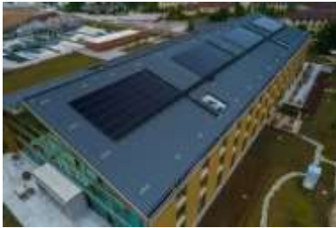
Zambelli RIB-ROOF_PV- Anlagen_05
