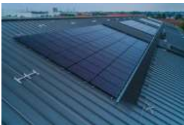
Zambelli RIB-ROOF_PV- Anlagen_07
